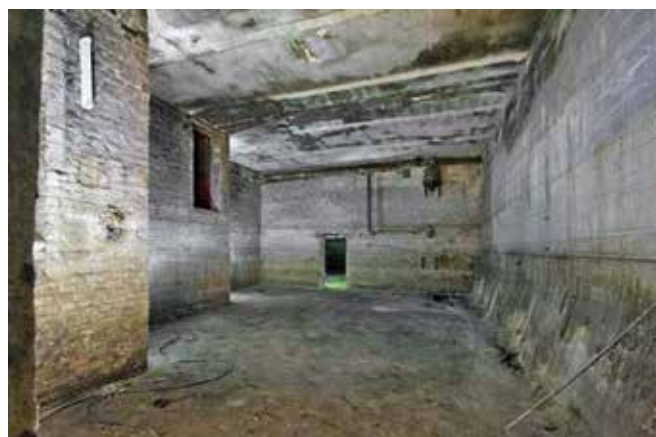
This room formerly divided into two floors, the ceiling level of the lower level is clearly seen as a line running round the wall. Note the ventilation equipment high on the far wall.
